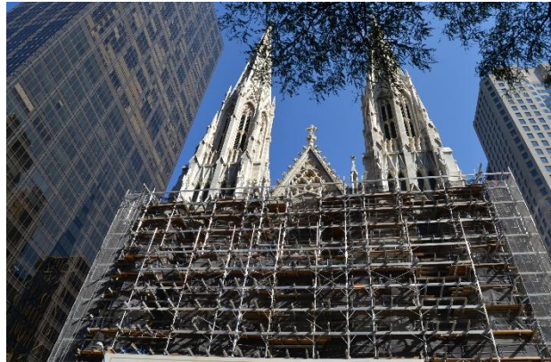
Figure 36: Saint Patrick's Cathedral under construction
