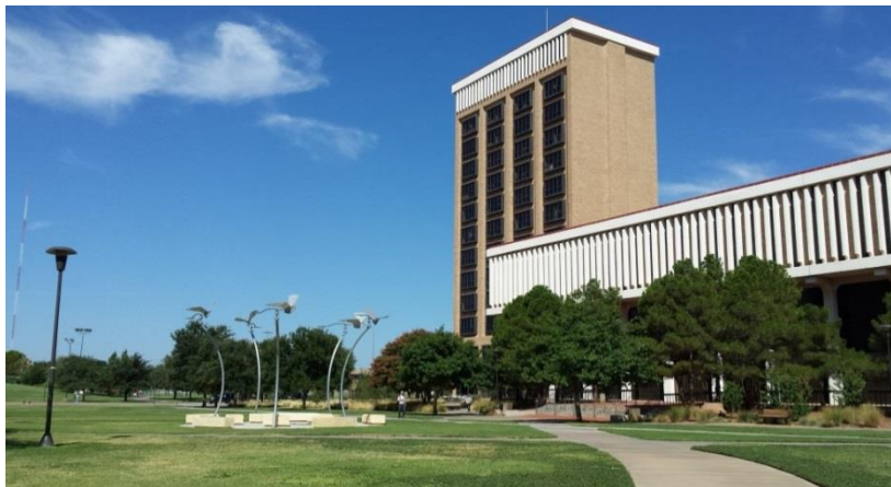
Figure 9: Back side of the library
