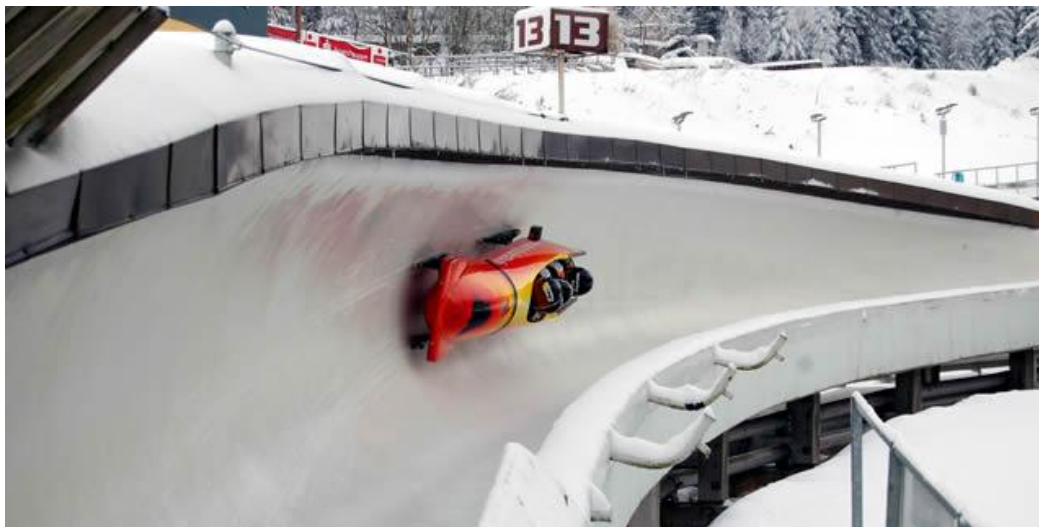
Abb. 6.1.1-2 Bobbahn in Altenberg 2
