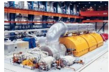
©: Siemens: Turbogenerator produced by Siemens, Germany.; CC BY-SA 3.0; 2005
