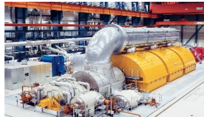
©: Siemens: Turbogenerator produced by Siemens, Germany.; CC BY-SA 3.0; 2005
