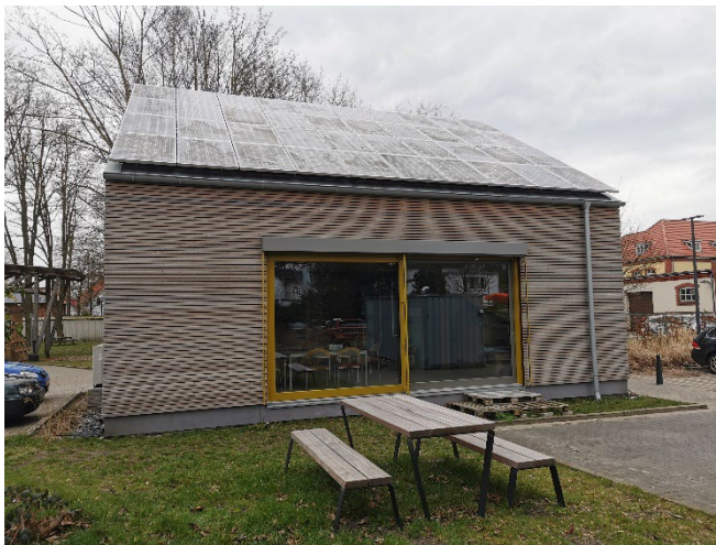
Figure 1: The energy efficiency test bench building
